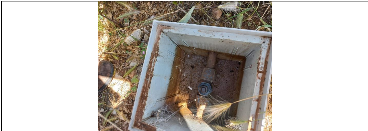
Figure 1.6: Existing pits for the installation of the ball tap valves
