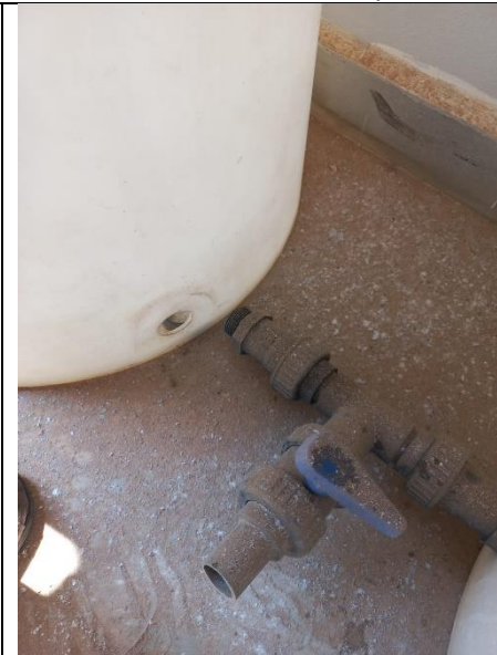
Figure 1.4: Connection between the two chlorination tanks
