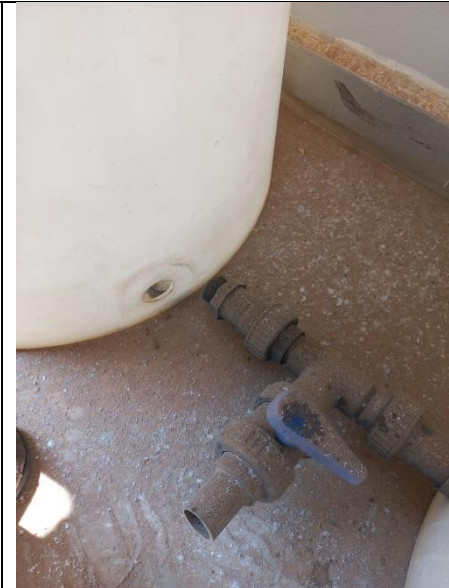
Figure 1.4: Connection between the two chlorination tanks
