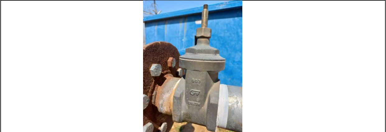
Figure 1.7: Existing 3 inches valve to be replaced
