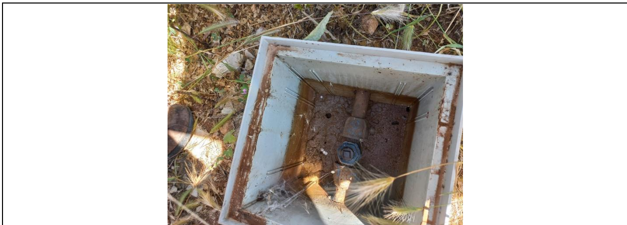
Figure 1.6: Existing pits for the installation of the ball tap valves
