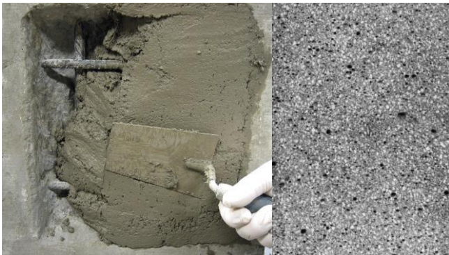
Figure 6. Hand applied mortar
