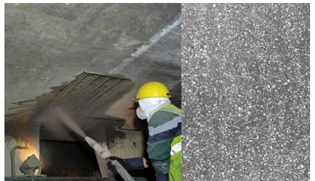
Figure 7 Maschine applied mortar. More densely packed.
