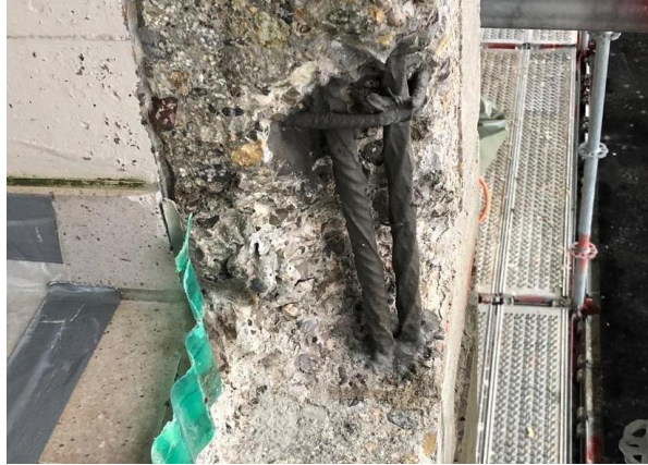
Figure 4. Applied corrosion protection SikaTop® Armatec®-110 EpoCem® on steel rebars
