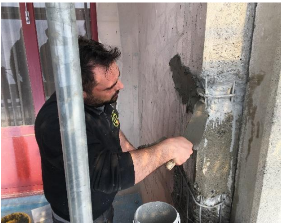
Figure 8. Hand application of repair mortar Sika MonoTop®-4012/ 12 Eco
