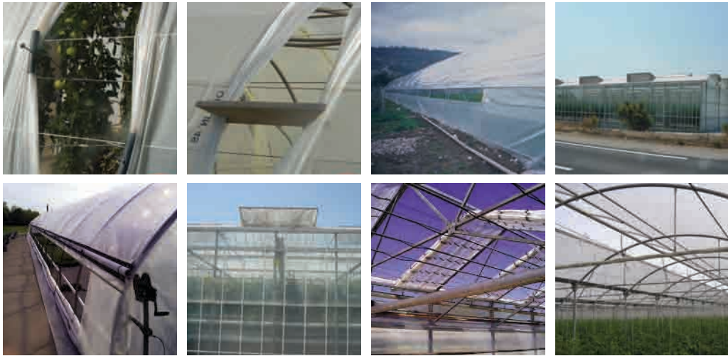
Plate 3 Different types of ventilation opening
