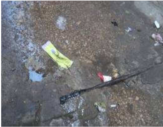
Leaking water supply pipes
