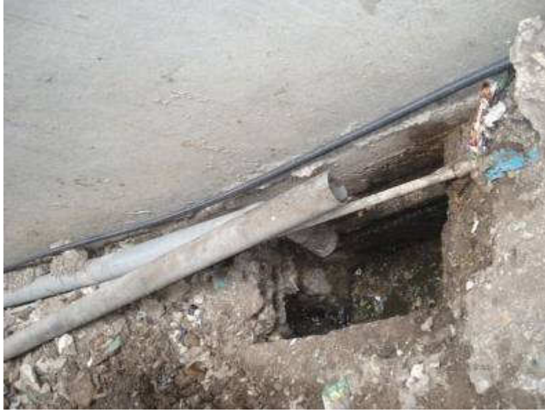
Uncovered inspection chamber, crossed by with water supply pipes
