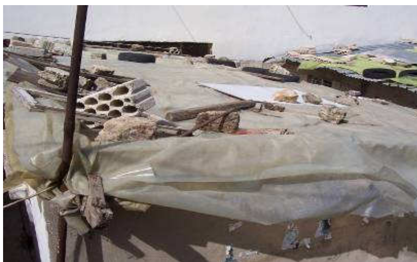
View of shelter zinc roof covered with plastic sheeting
