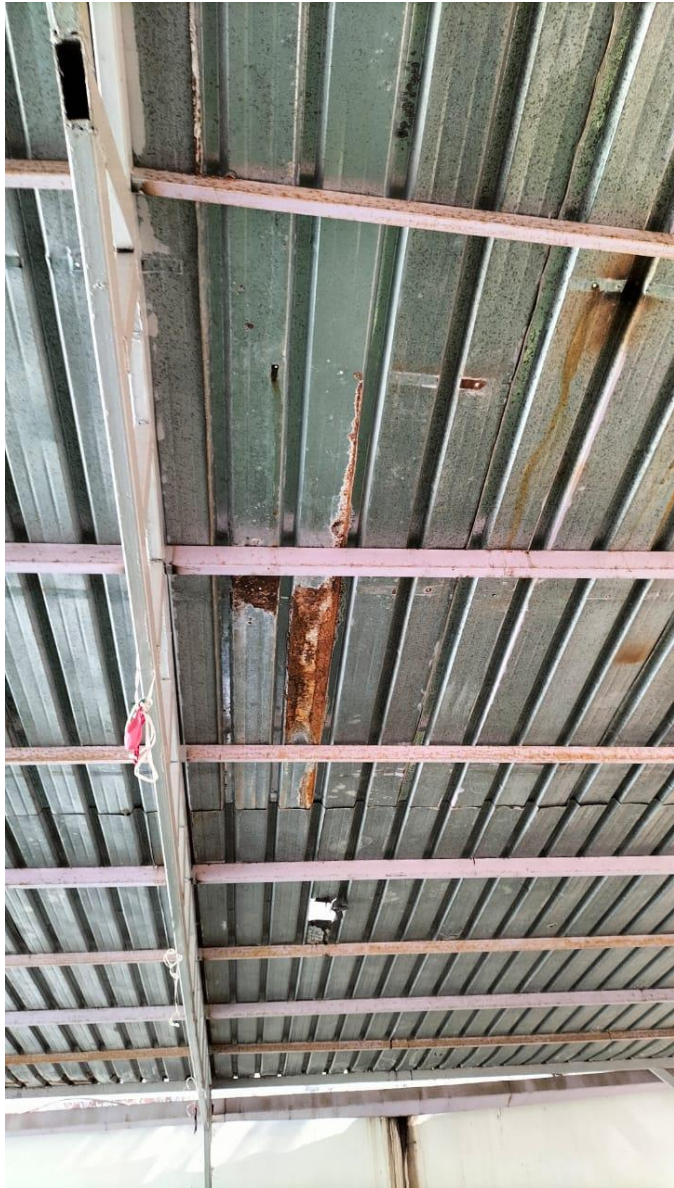
Photo 3-Rusted Zink Roof
