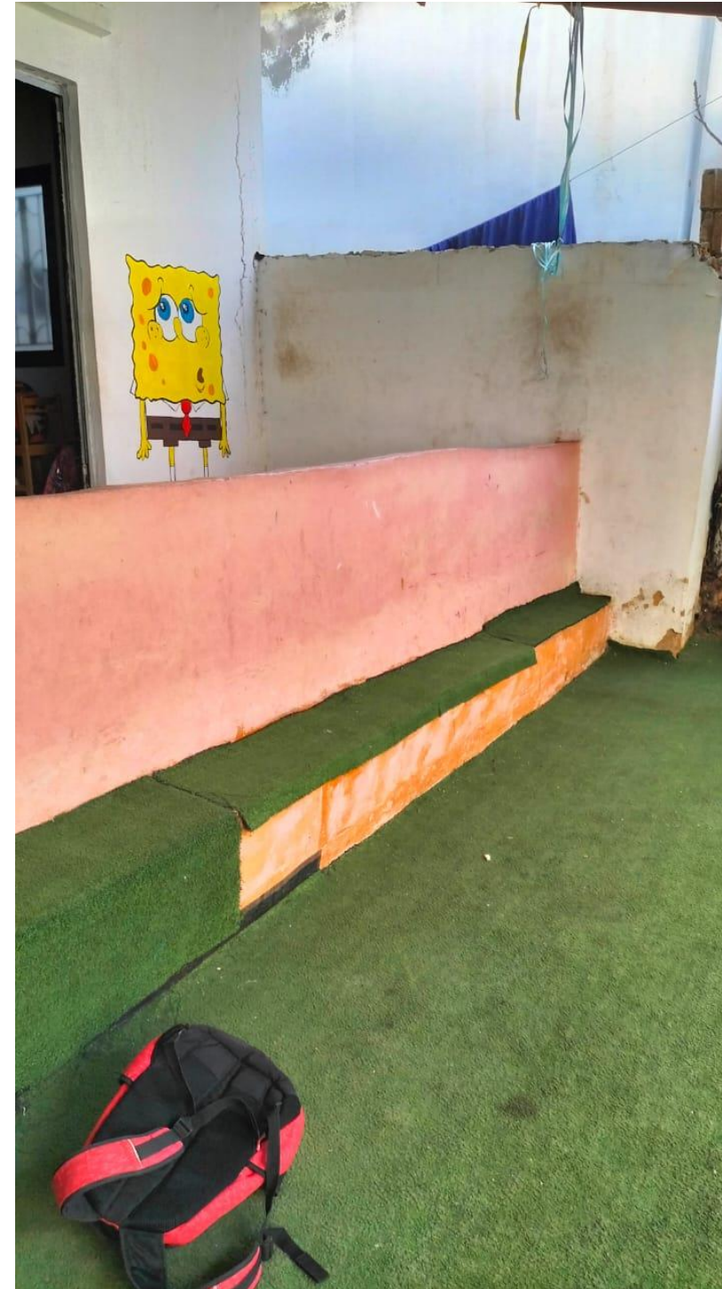
Photo 4- Artificial grass removed in the seating area
