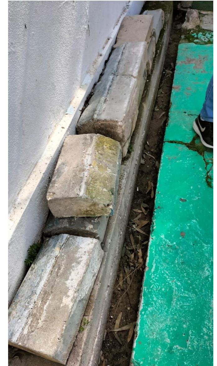
Photo 2- Uncovered Water channel
