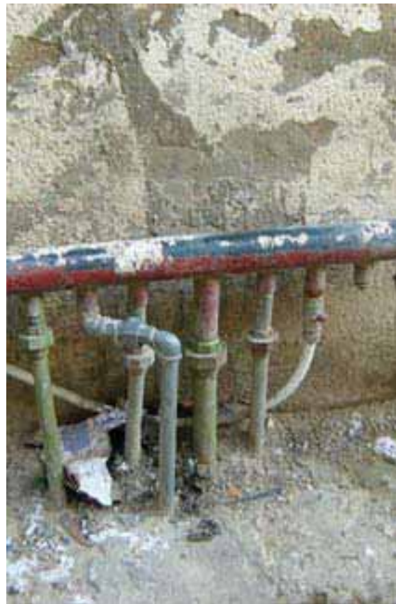
Collective water manifold installed by dwellers in Bustan about Jamil
