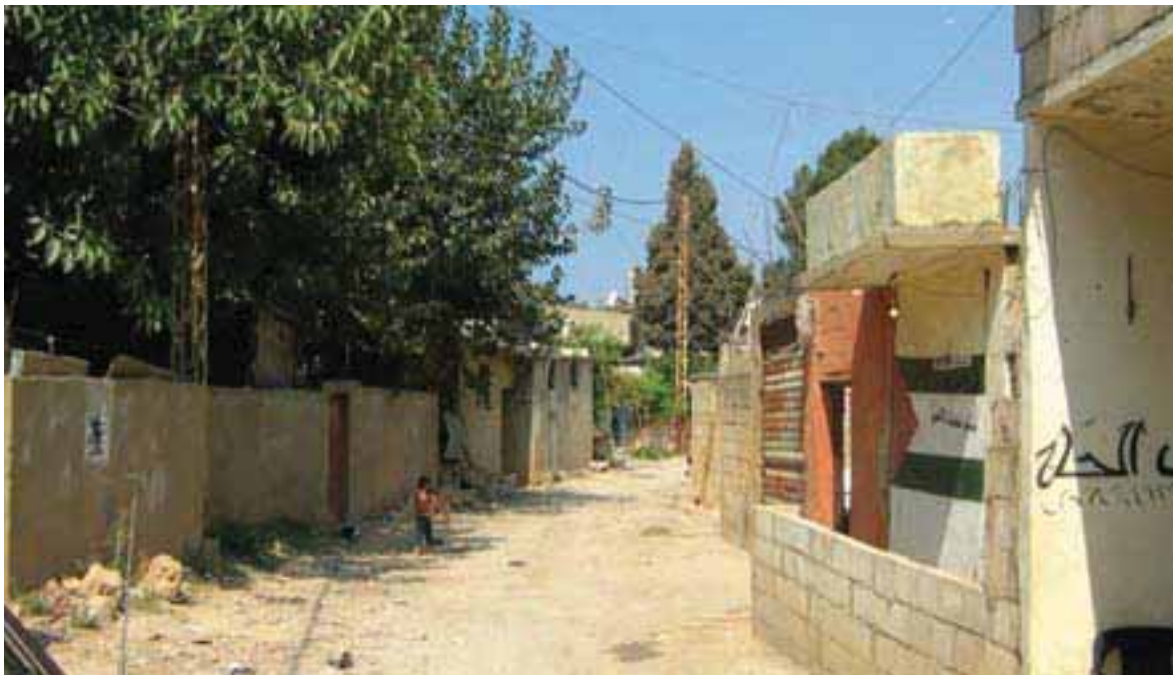
EDL provides electricity in some informal settlements in Lebanon, as shown in the AA of Tallet el Mankoubin around Beddawi Camp in North Lebanon
