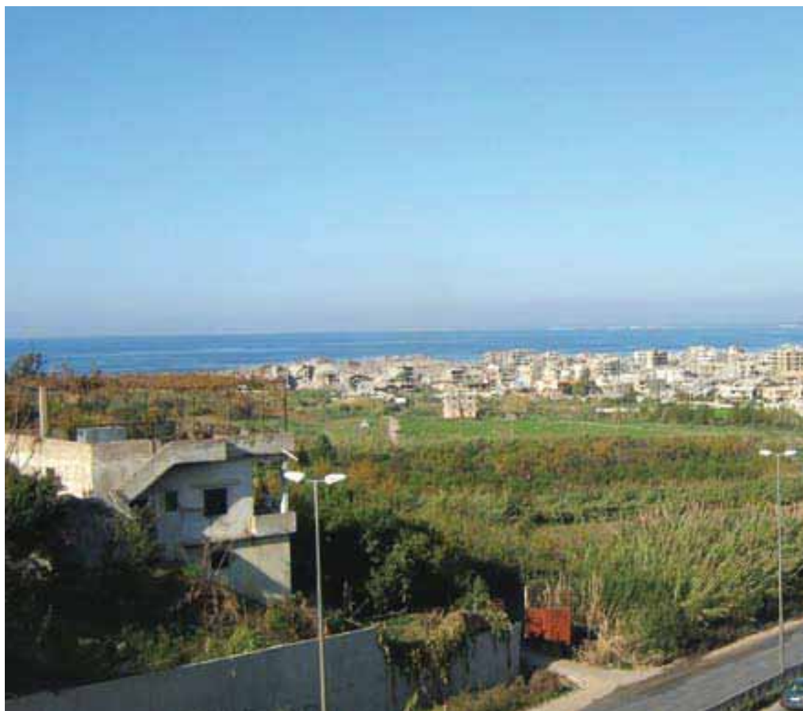
The destroyed Nahr el Bared Camp surrounded by the extended Adjacent Area (Source NBRC)
