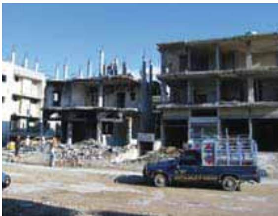
Relief works undertaken by UNRWA and other agencies in NBC AA after 2007 conflict (Source NBRC)
