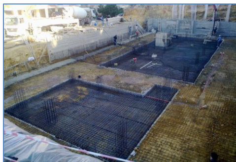
December 2010 - The Foundations
