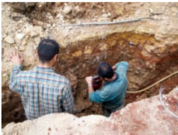
◀ Repair of Water Conduits in Borj Al Barajneh
