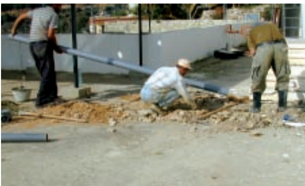
◀ Kfar Hamam: Rehabilitation of Municipality sewage system.
