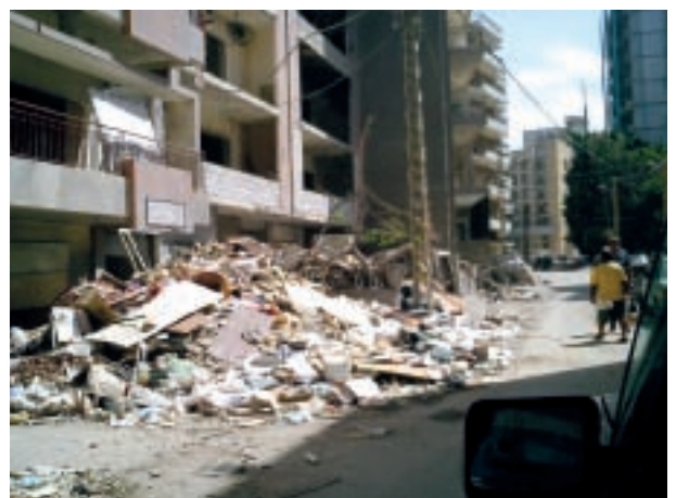
▲ Destruction in Maawad Area
