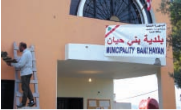
▲ Beni Haiyane: Restoration and rehabilitation of the Municipality premise
