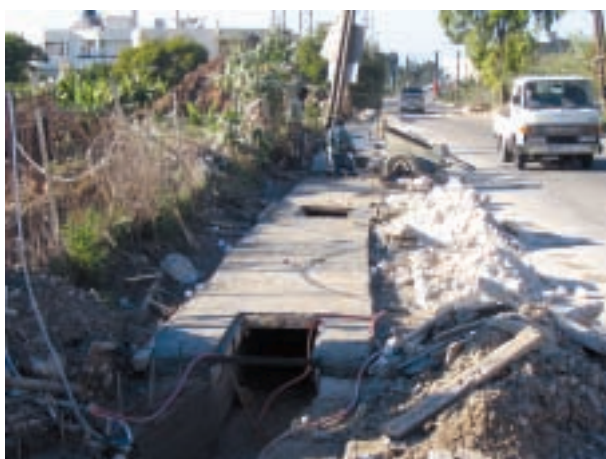
◀ Charqieh Store Water Conduits
