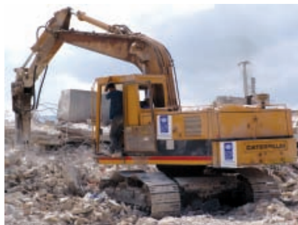
▲ Rubble Removal in Qana
