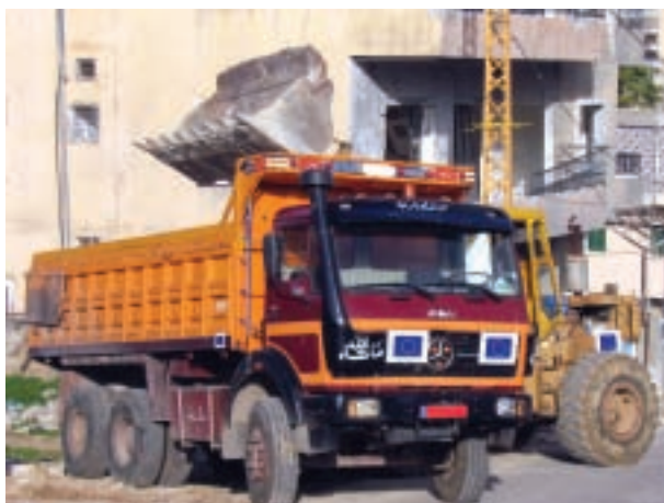
▲ Rubble Removal in Nabatieh
