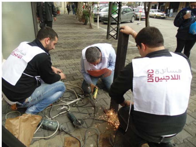
Road rehabilitation Community Support Project (CSP), North Lebanon, October 2013
