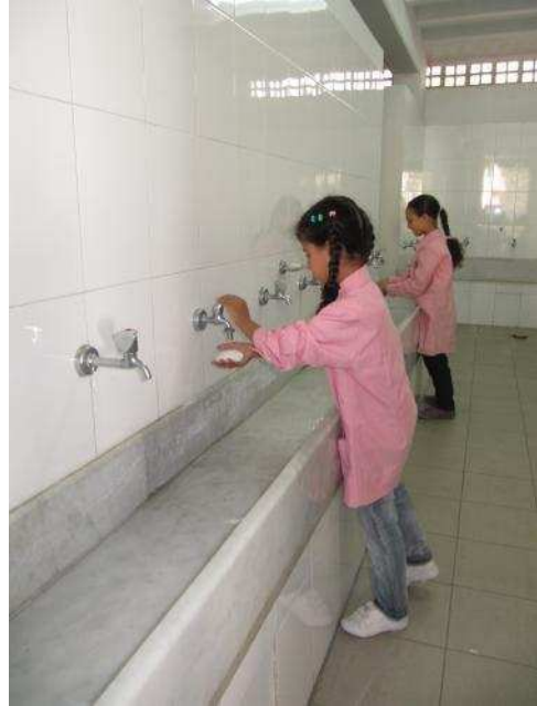
Adequate Wash basins
