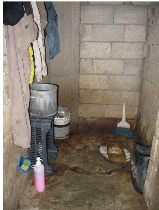
Toilet to be maintained
