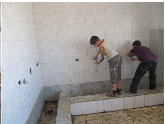
Inadequate drinking facilities
