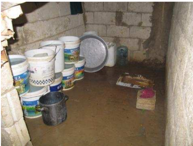
Toilet to be maintained
