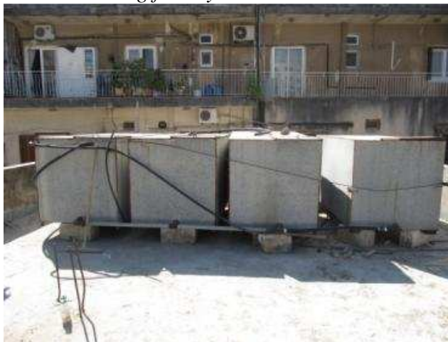
Water tanks to be replaced
