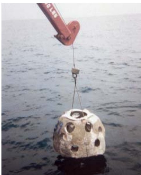
Figure 7.10. Rubble and Prefabricated Concrete Material used for AR Construction
