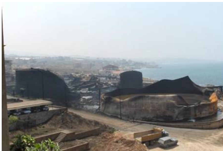
Figure 4.4. The Fuel Tanks after the Fire Consumed the Stored Fuels
